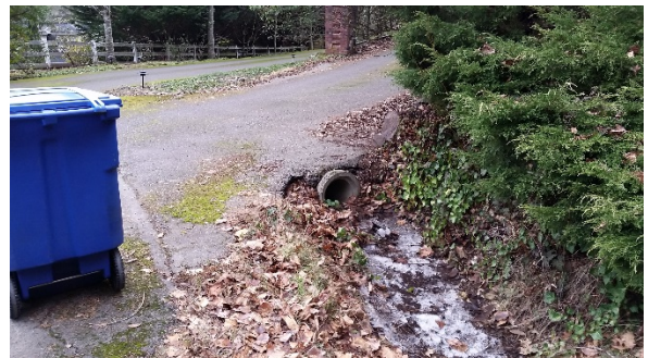
8 – Looking southwest at 12-inch culvert pipe
