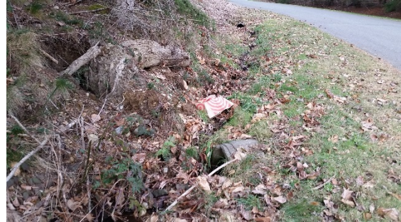
6 – Looking northeast at outlet end of 12-inch culvert pipe running underneath 222 nd PI SE
