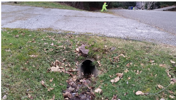
3 – Looking at 12-inch culvert pipe
